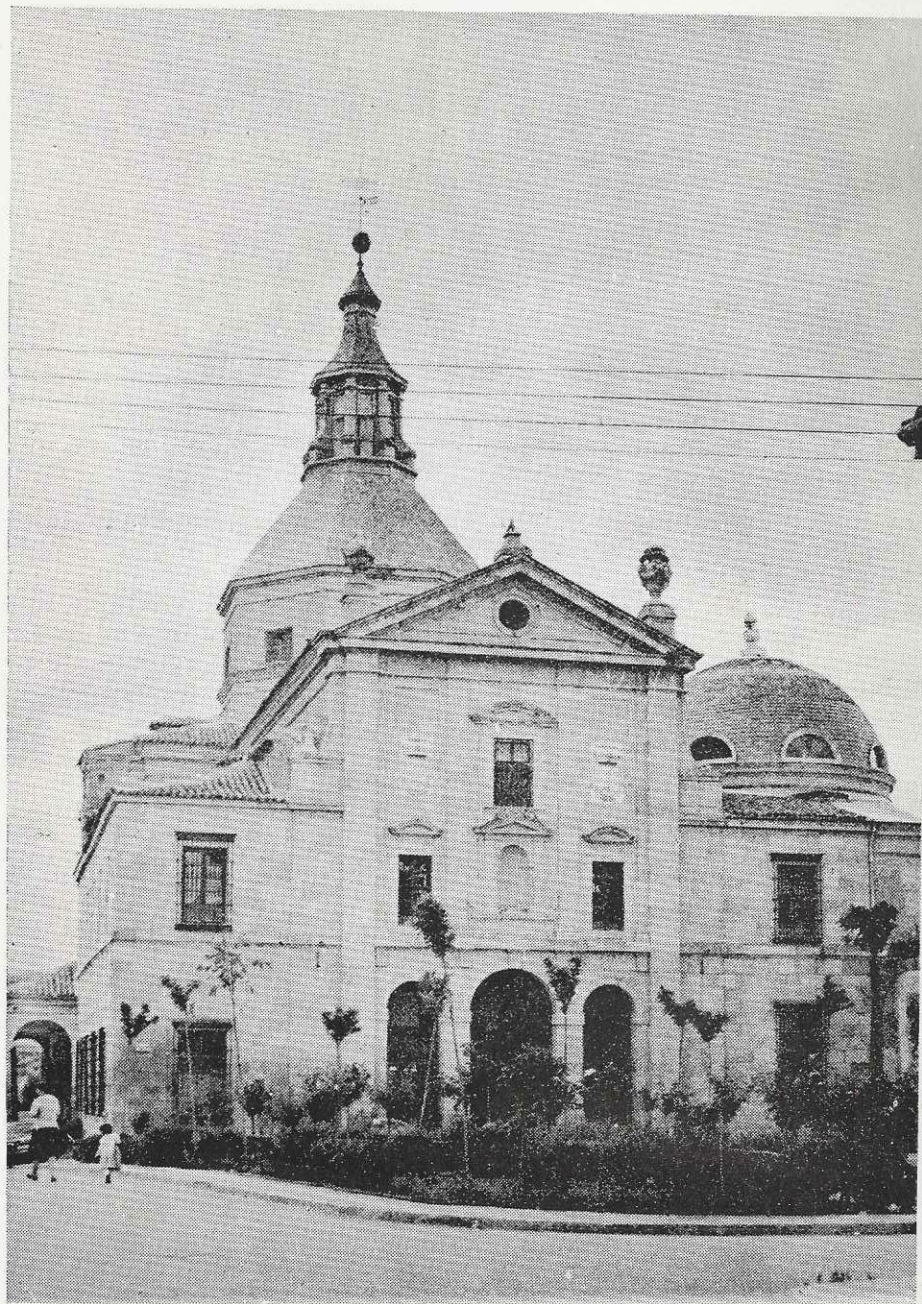
Fachada principal Convento Dominicas
